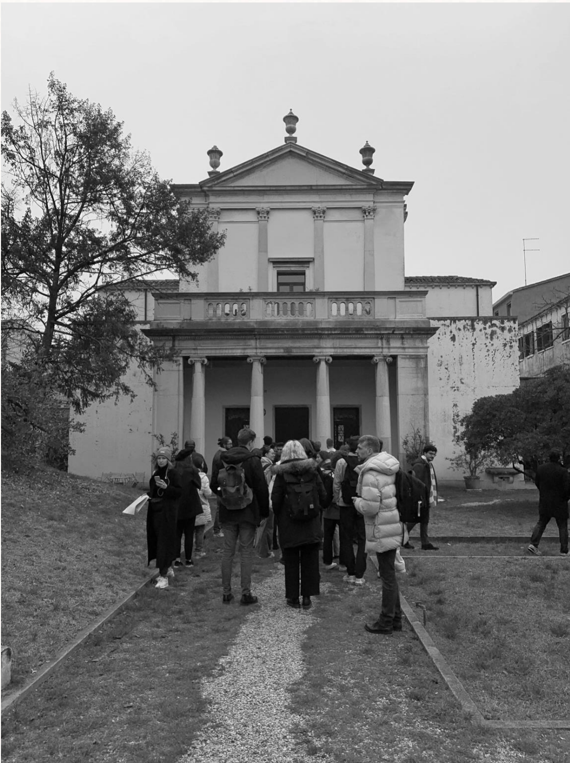
The view of the Neoclassical Loggia. Source: Photograph taken by the author.
