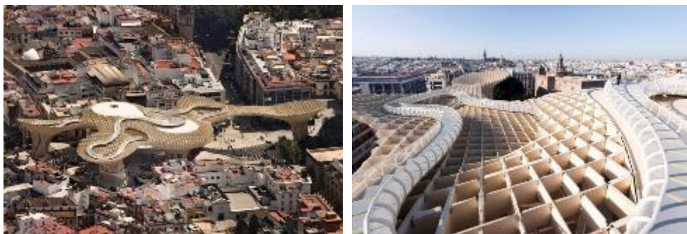
Figure 1. Complex wooden structure - Metropol Parasol in Seville, Spain, (Cilento, 2012)
