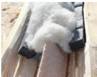
Figure 8. Composite strip - wool fleece and memory foam between logs (house No.3)
