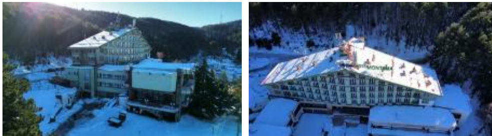
Figure 1. Photos from Hotel Montana – Existing Condition (private photos)
