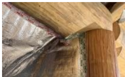
Figure 4. Membrane sealed to post/beam
