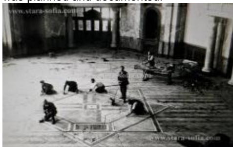
Figure 2a: A moment from the construction of the Rectorate of Sofia University - craftsmen laying the parquet floor in the Aula, early 1930s. Archive photos. Old Sofia ( www.stara-sofia.bg )
