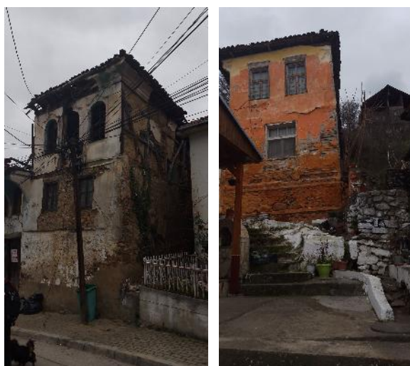
Figure 1. Selected Timber structures in the city of Strumica (current state)
