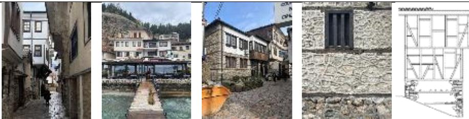
*Figure 1. The Ottoman Era Houses in Ohrid, Macedonia – the wooden structural system (bondruk system) of the traditional Macedonian house*
