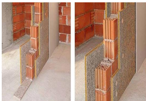
Figure 6. The application of heraklith panel with stone wool core.
