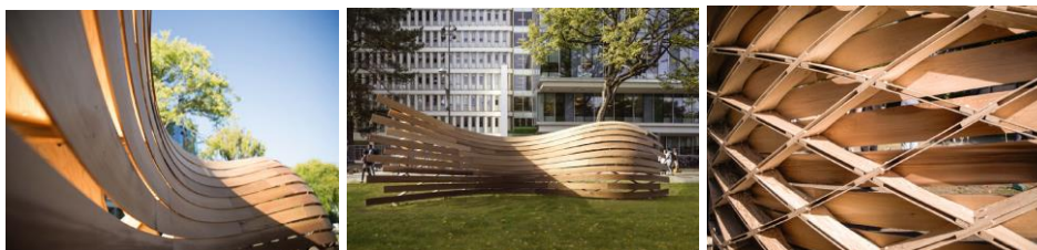
Figure 3. Wooden structures as a product of digital design and implementation: Timber Wave prototype, doubly curved timber assembly, at the University of British Columbia Campus [3].
