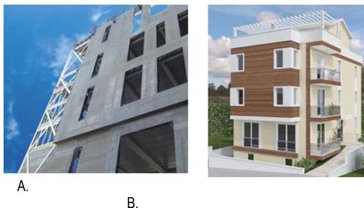
Figure 3. A. Cement bonded particleboard for Sheathing of walls and partitions.
