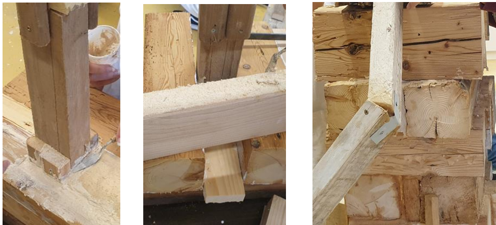
Figure 4.5.6. Sawdust and glue putty, joining beams, small beams and slats, various sizes and types of wood
