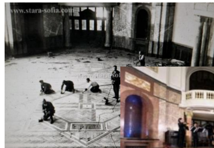
A moment from the construction of the Rectorate of Sofia University - craftsmen laying the parquet floor in the Aula, early 1930s.
