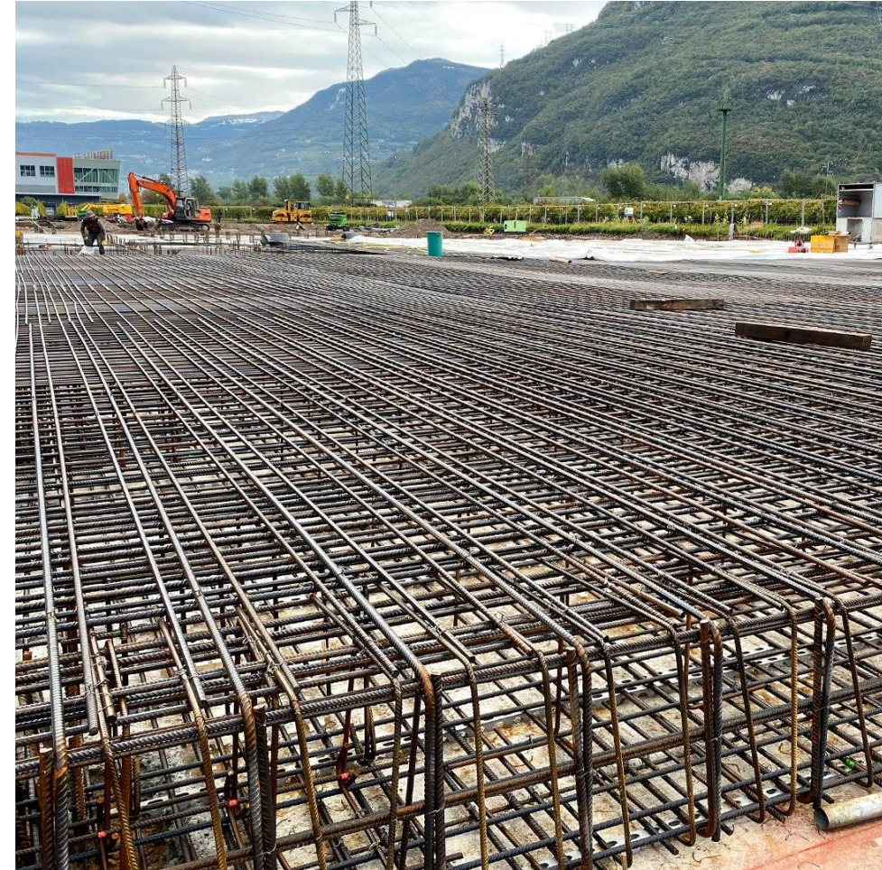
The massive slab was tied to the pilings, a structural rebar grid added, and concrete poured.
