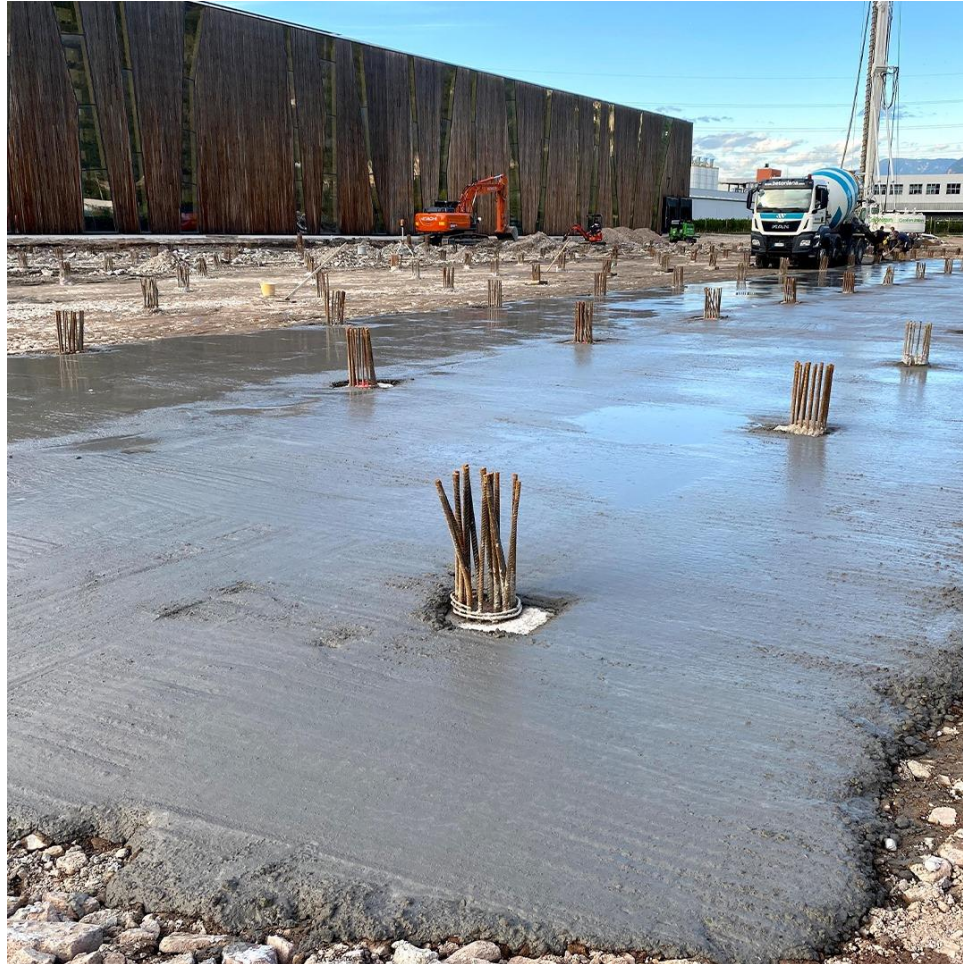
The massive slab was tied to the pilings, a structural rebar grid added, and concrete poured.
