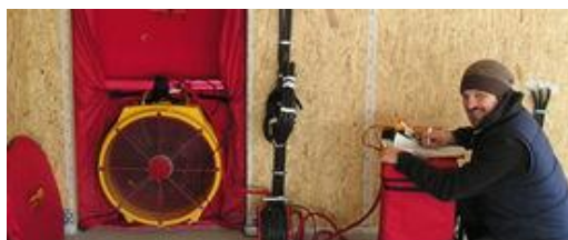
Figure 4. Blower Door Test being conducted in a house with OSB4 as main air barrier
