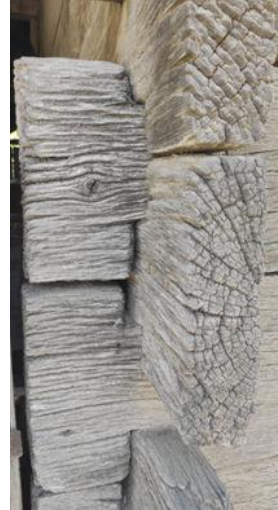
Figure 4. "Croatian" joint, Čigoč
