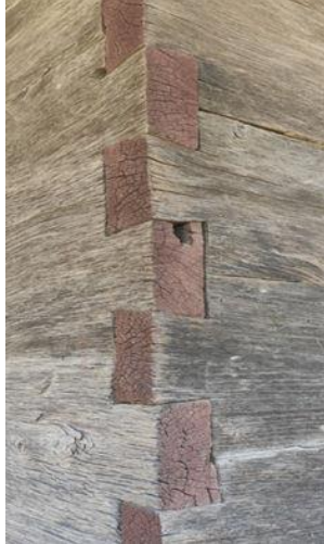
Figure 3. "German" joint, Čigoč
