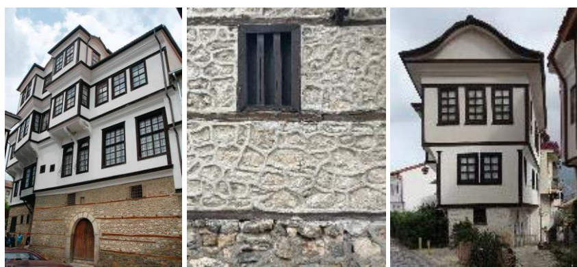
Figure 2. The Ottoman Era Houses in Ohrid, Macedonia – the wooden structural system (bondruk system) of the traditional Macedonian house
