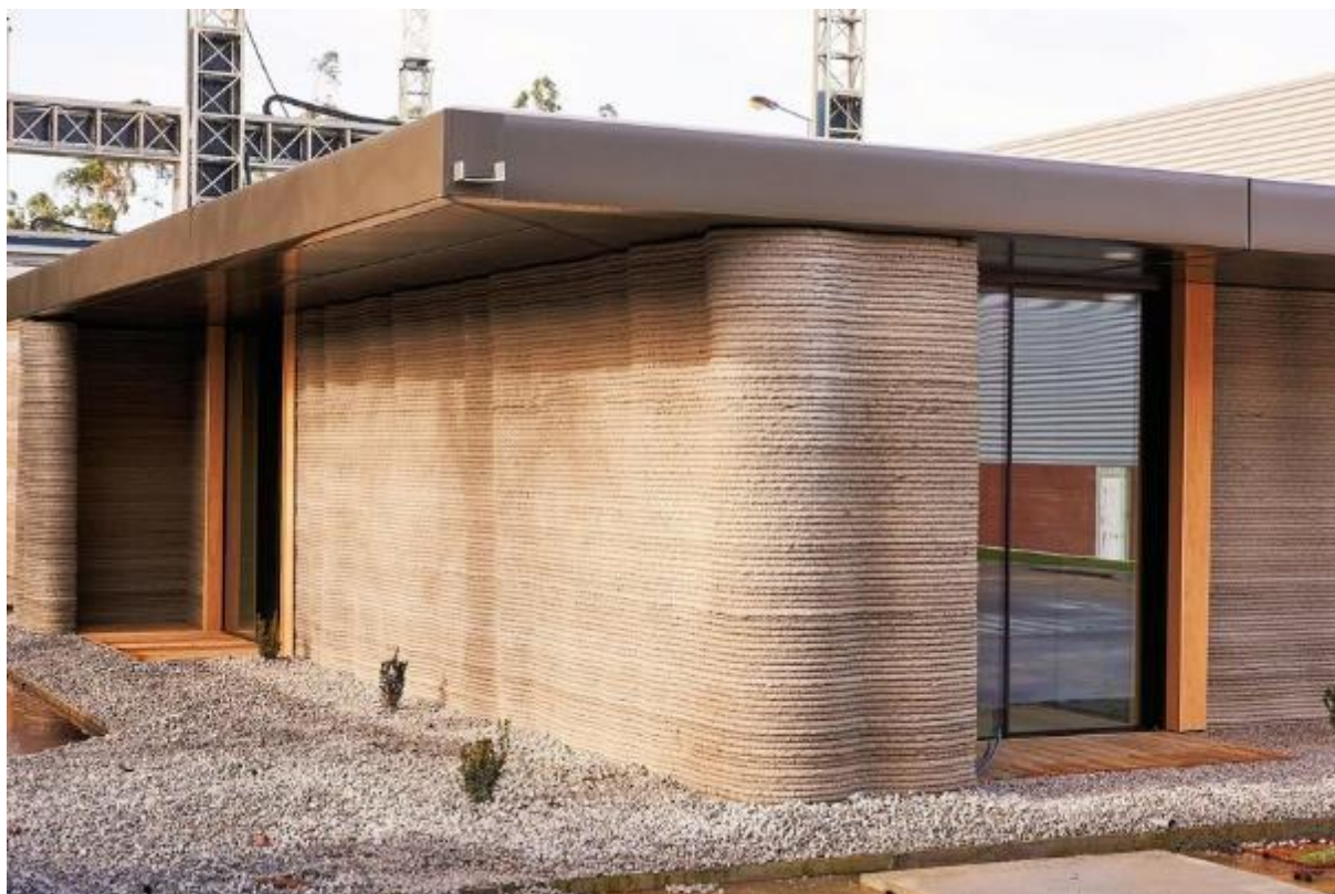
Figure 5. House made of wooden recycled material by 3D printing ( https://constructive-voices.com/sk/7-kr%C3%A1snych-3D-tla%C4%8Den%C3%BDch-domov/ )
